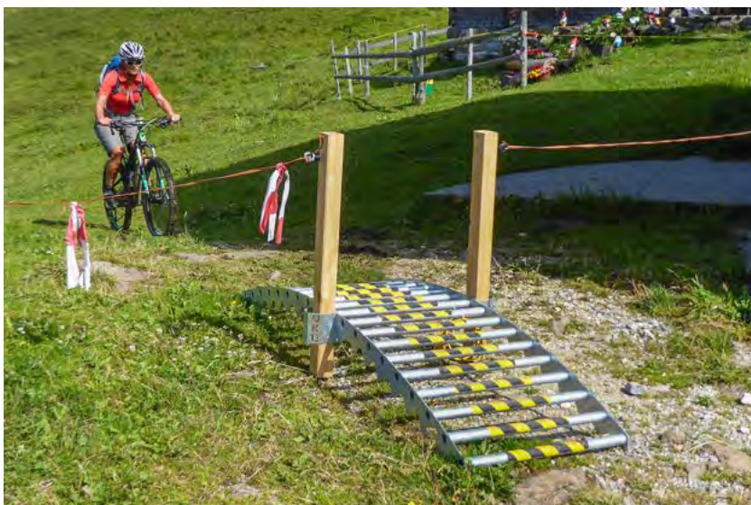
Fig. 94 Rampa ad arco transitabile in mountain bike
